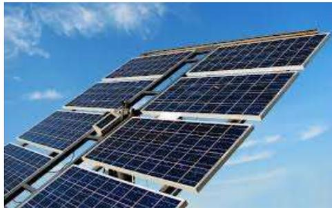
Electrical connections are made in series to achieve a desired output voltage and/or in parallel to provide a desired amount of current source capability. Diodes are included to avoid overheating of cells in case of partial shading. Since cell heating reduces the operating efficiency it is desirable to minimize the heating hence to provide good ventilation behind the module.
