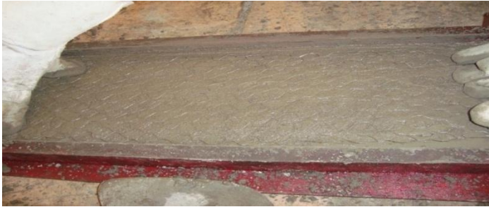
Figure 3.13 Placing of steel wire mesh
