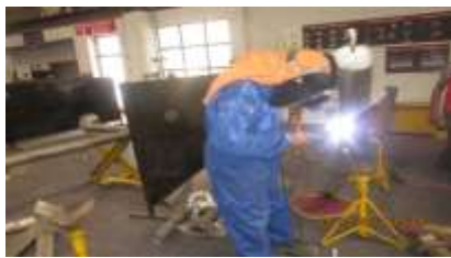
Fig.1. Welding in awkward postures on one side of the pipe
