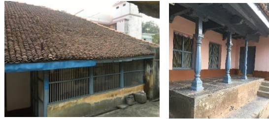
Figure 5 Shaded windows with roof Projections
